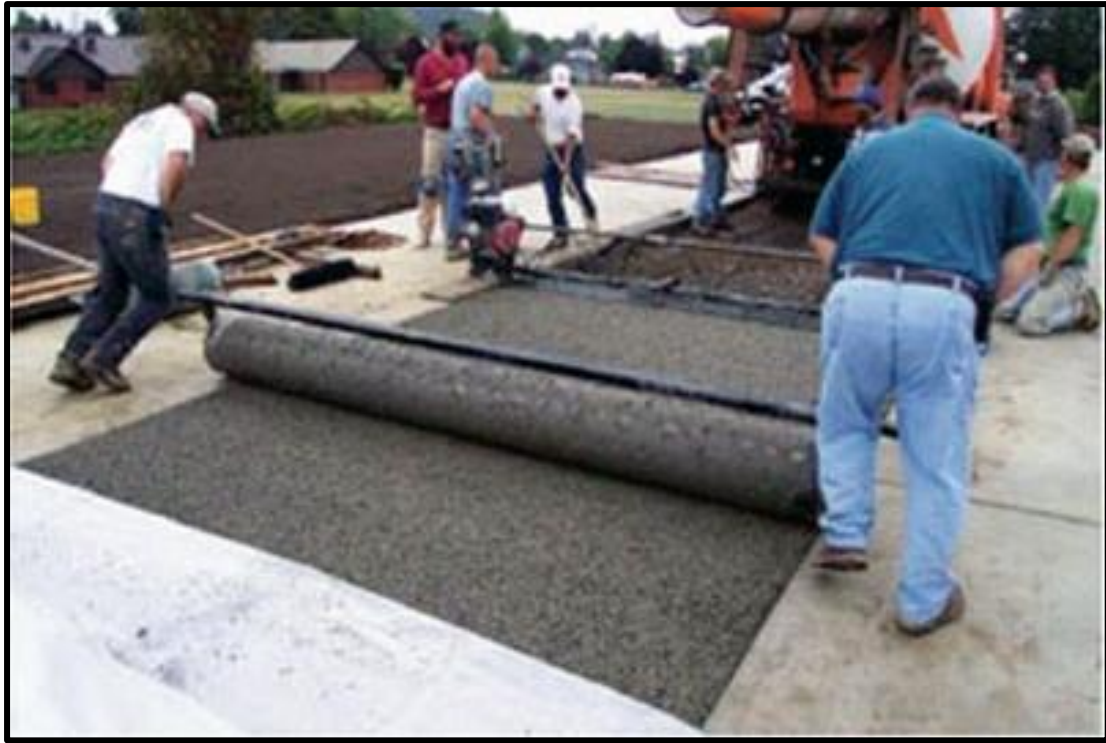
Figure 1.4 Pervious concrete compaction (NRMCA, 2011)
