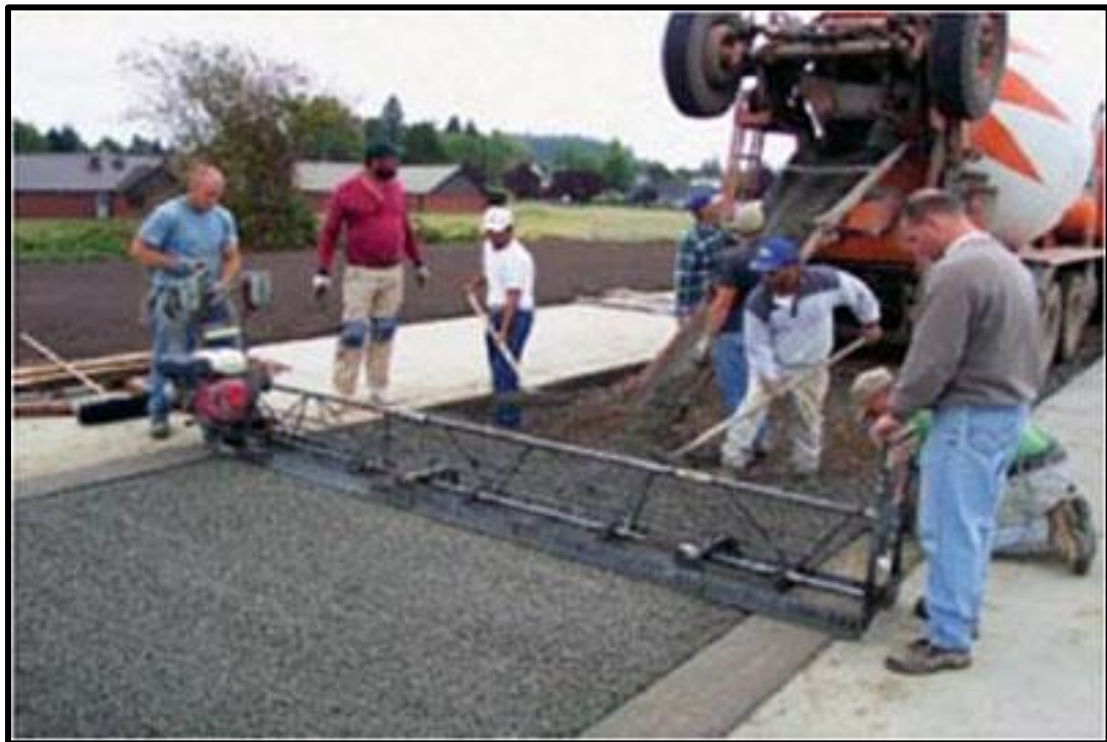
Figure 1.3 Pervious concrete placement (NRMCA, 2011)
