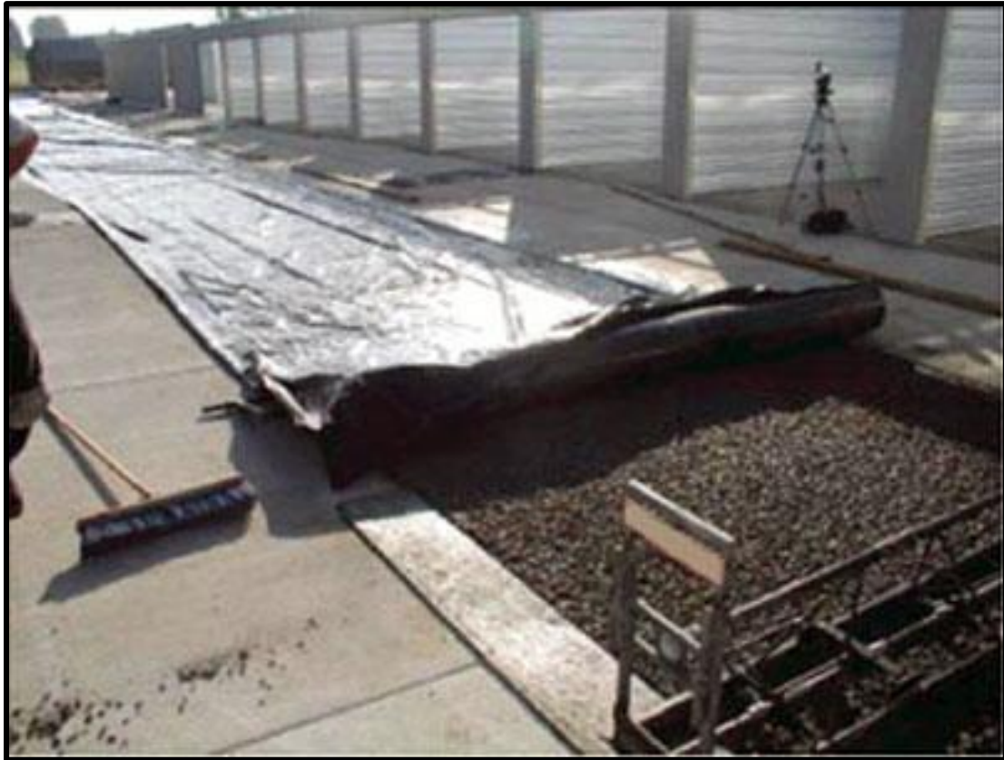
Figure 1.5: Pervious concrete curing by plastic sheeting (NRMCA, 2011)
